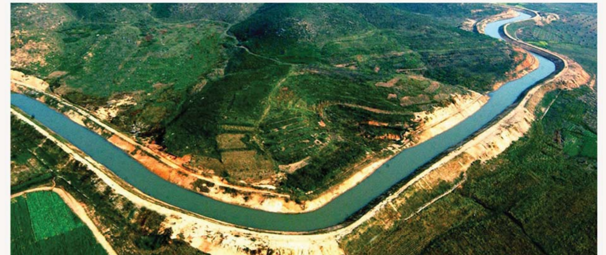
Gravitational waterways and fish and stockbreeding farms are built
